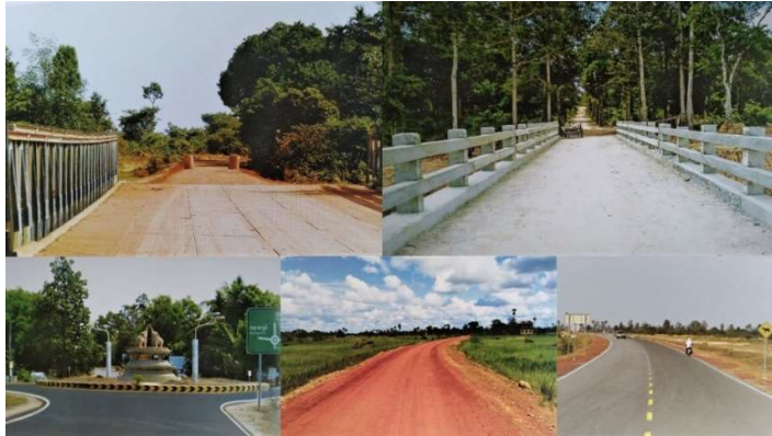
Picture 5.5.1 (B) Road and bridge constructions
