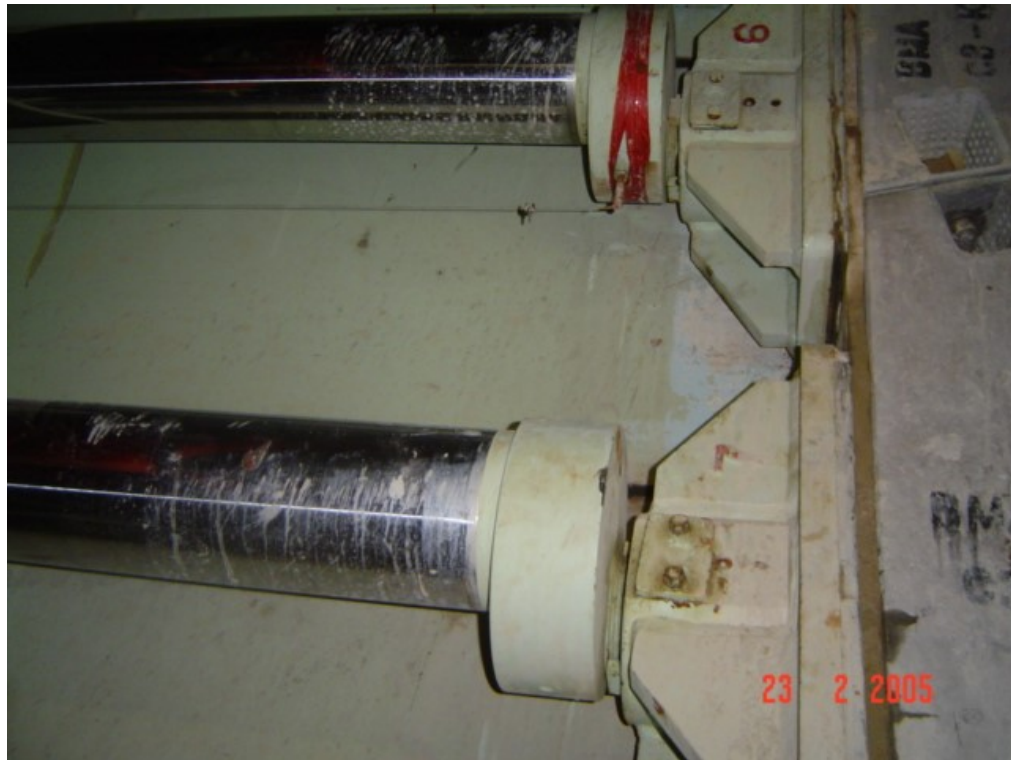
Figure 2.10 Hydraulic jacks pushing on the segmental lining behind the shield (BMA flood diversion project, Saensaep-Latphrao Phrakhanong)
