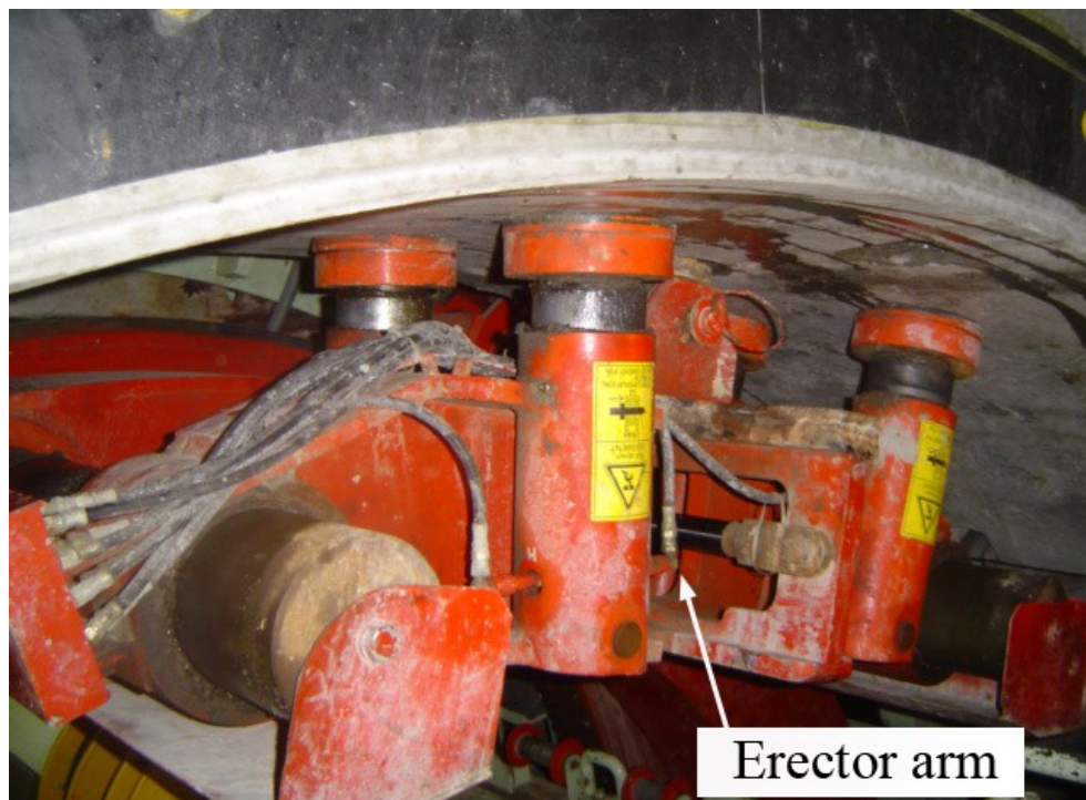
Figure 2.12 Erector arm installing a segmental lining at the crown of the tunnel (BMA flood diversion project, Saensaep-Latphrao Phrakhanong)
