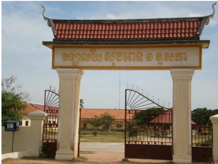
Picture 3.2 School and classroom built by members of the CPP, Cambodia
